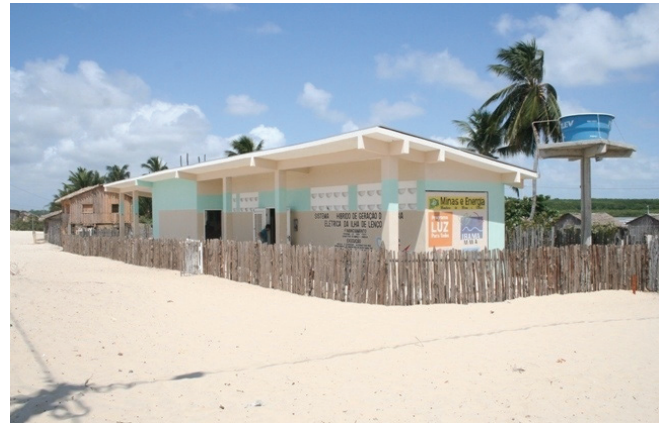
Fig. 6 Control and power house.
