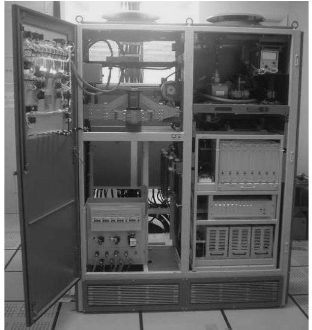
Fig. 9. Atlas radar transmitter after upgrade
